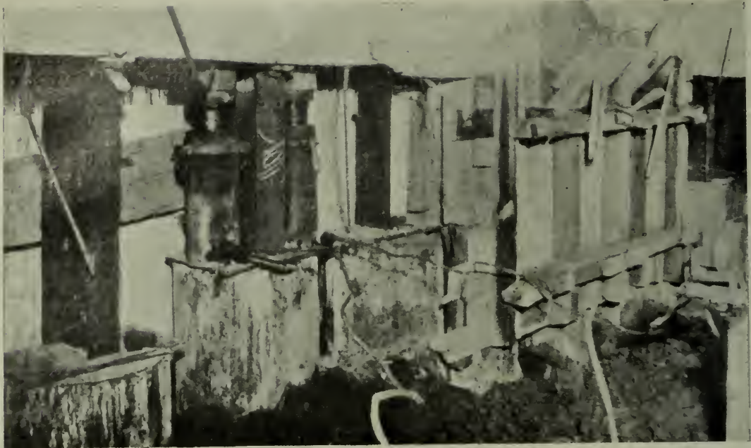
FIG. 6. TESTING "PRETEST" PILES UNDER EXTERIOR WALLS.
